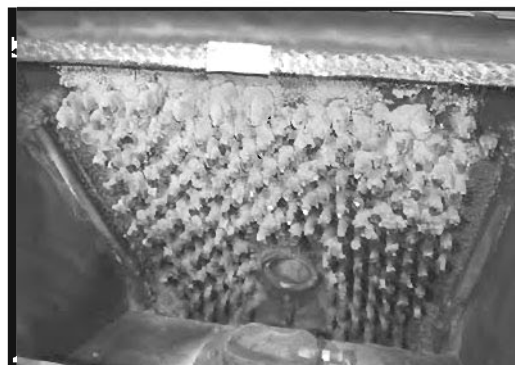
Figure 17.2 - Example of a dirty heat exchanger
