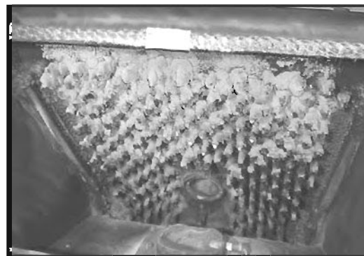
Figure 17.2 - Example of a dirty heat exchanger
